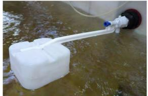
Fig. 9.11 Ballcock & Float Valve Controlling the Water in the Sump Tank
