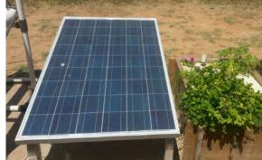
Fig. 9.7 Photovoltaic Cells Used to Power a Water Pump
